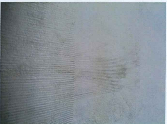
Image 5: Completed TOUR-quality rake job.
